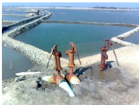
Photograph 6.6: Hand tube-wells on the embankment caused damages
