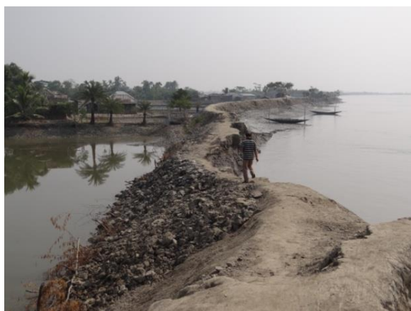
Photograph 6.3: Worst condition of embankment near Maider char
