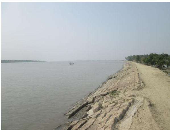
Photograph 5.2: Deteriorated Condition of Existing Slope Protection Work
