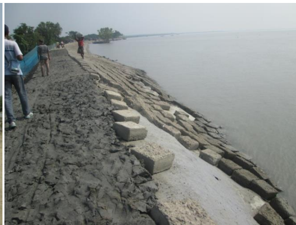
Photograph 5.2: Deteriorated Condition of Existing Slope Protection Work
