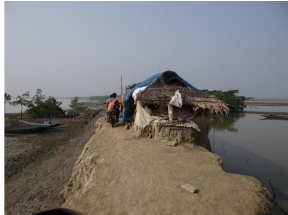
Photograph 6.4: Vulnerable condition of embankment near Jalakhali
