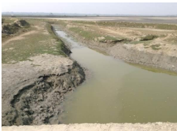
Photograph 6.5: Deteriorated drainage khal in D/S-2 and D/S-1
