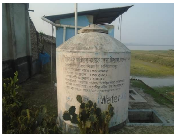
Photograph 6.28: Drinking water filtering system in the Polder
