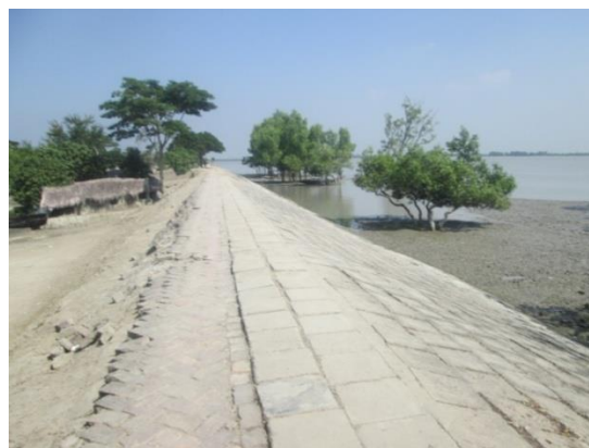
Photo 5-4: Present condition of existing slope protection work
