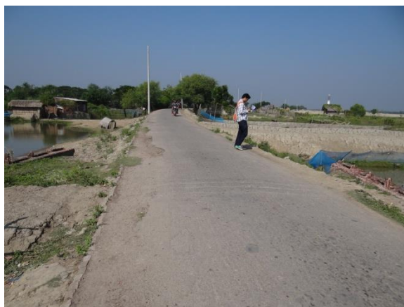
Photo 5-3: Bitumen carpeting on the crest of the embankment
