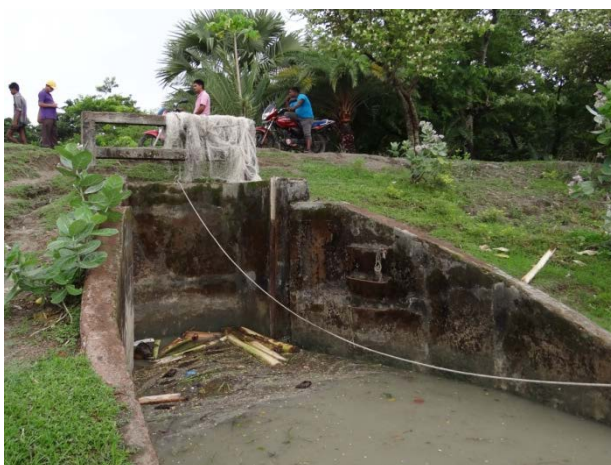
Non-Functioned Drainage Sluice (DS1)
