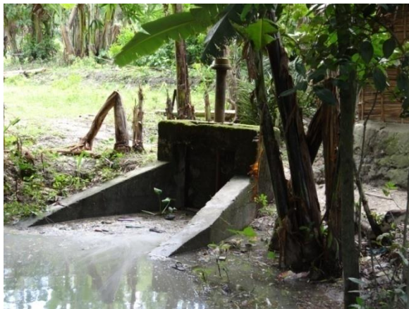
Picture 5: Non-functioning Flashing Sluice( FS5)
