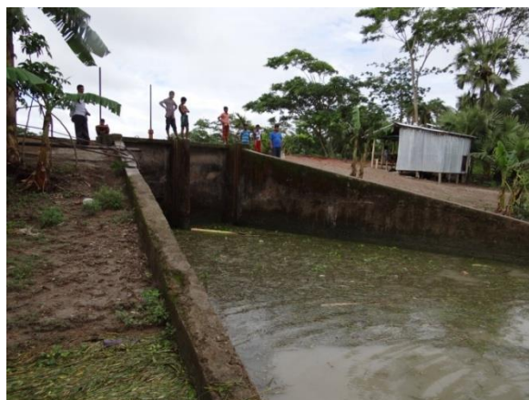
Picture 1: Non-function Drainage Sluice (DS6)
