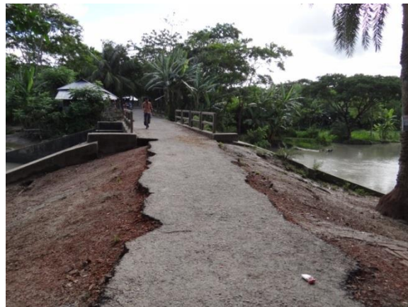
Picture 6: Breached embankment
