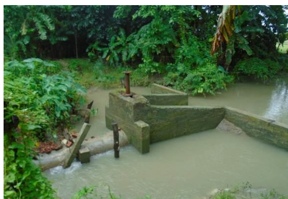
Picture4.10: FS-1 (1V-0.9m dia) Flushing Sluice at Char Shuhari on Shuhari Khal (Ch. 25.20 km)
