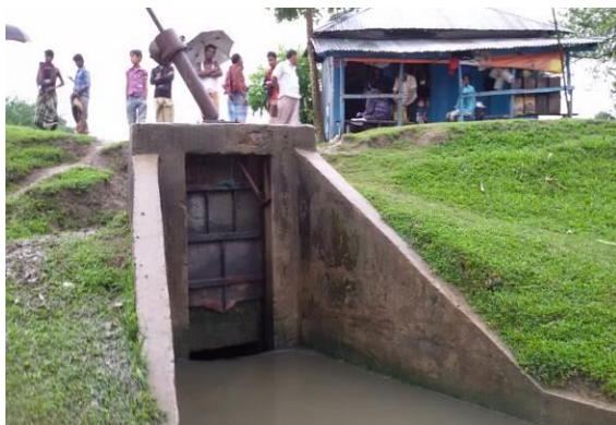
Picture4.8: DS-5 (1V-0.9m X 1.2m) Sluice at Alir Bazar on Pollar Khal (Ch. 8.34 km)
