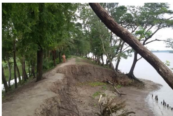
Picture 4.14: Worst embankment at Ch. 13.20 km to 14.0 km
