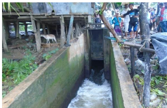
Picture 4.6: DS-3 (1V-0.9m X 1.2m) Sluice at WAPDA Boderhut on Golkhali khal (Ch. 17.50 km)
