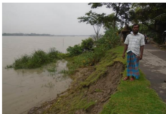
Picture 4.15: River bank erosion at Ch. 19.20 km to 19.70 km
