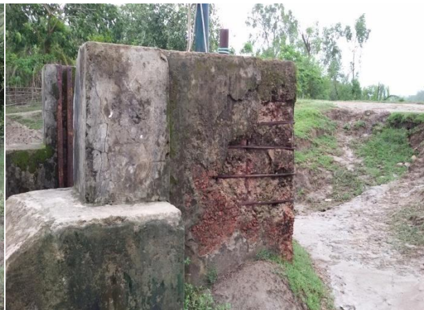
Picture 2: Damaged Drainage Sluice (DS2)
