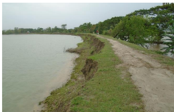
Picture 5.13: River bank erosion at Payerpur Ch. 2+550 km (21°53'51.6" N; 90°9'26.3" E, Date: 23 July 2015)
