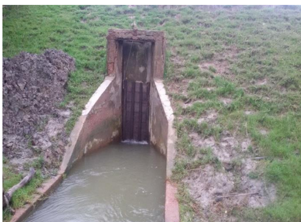
Picture 5: Non-functioned Flashing Sluice (FS)
