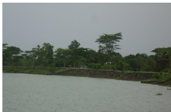
Picture 5.13: River bank erosion at Payerpur Ch. 2+550 km (21°53'51.6" N; 90°9'26.3" E, Date: 23 July 2015)
