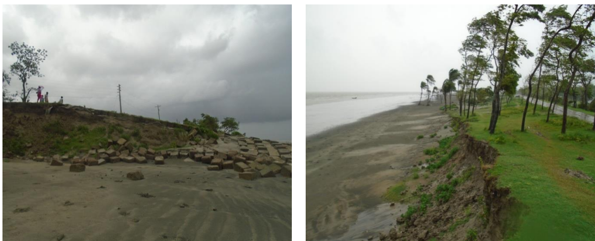
Picture 4.2: Deteriorated condition of bank protection (Kuakata sea beach)
