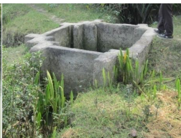
Photograph 5.7 : Flushing sluice at Lashmi khali
