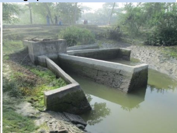
Photograph 5.3 : Flushing sluice at Gomoti
