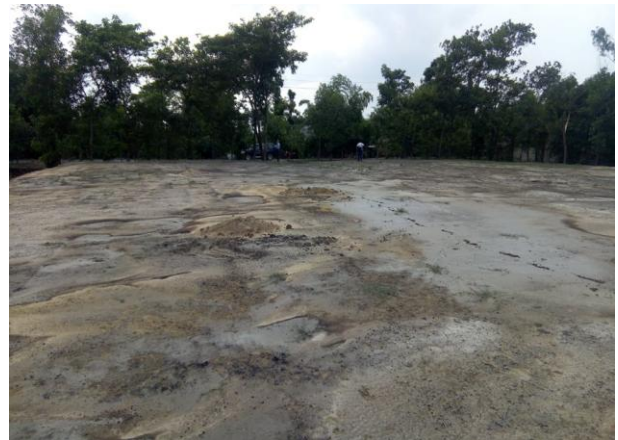
FIGURE 9: THE SUBSTATION SITE HAS BEEN RAISED ABOUT 5 FEET HIGH BY FILLING EARTH MATERIAL
