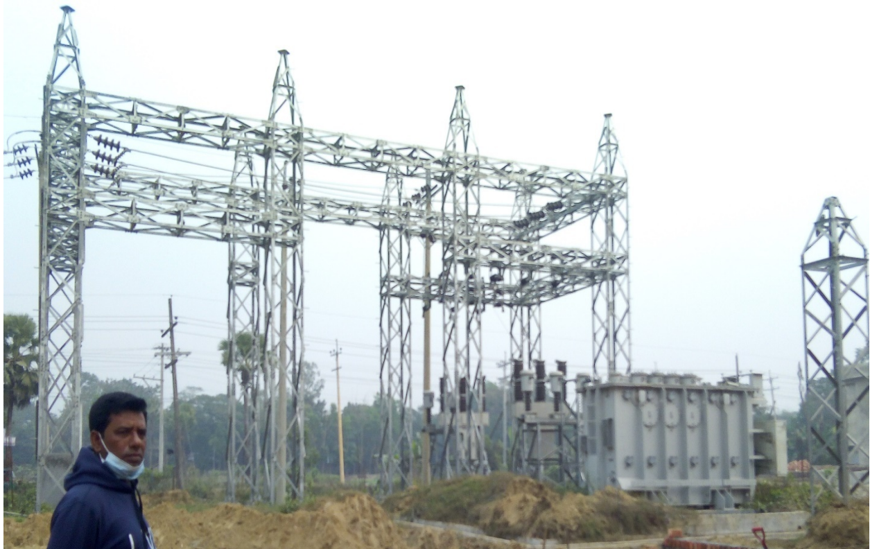
FIGURE 5: OUTDOOR COMPONENTS OF AN ELECTRICAL SUBSTATION
