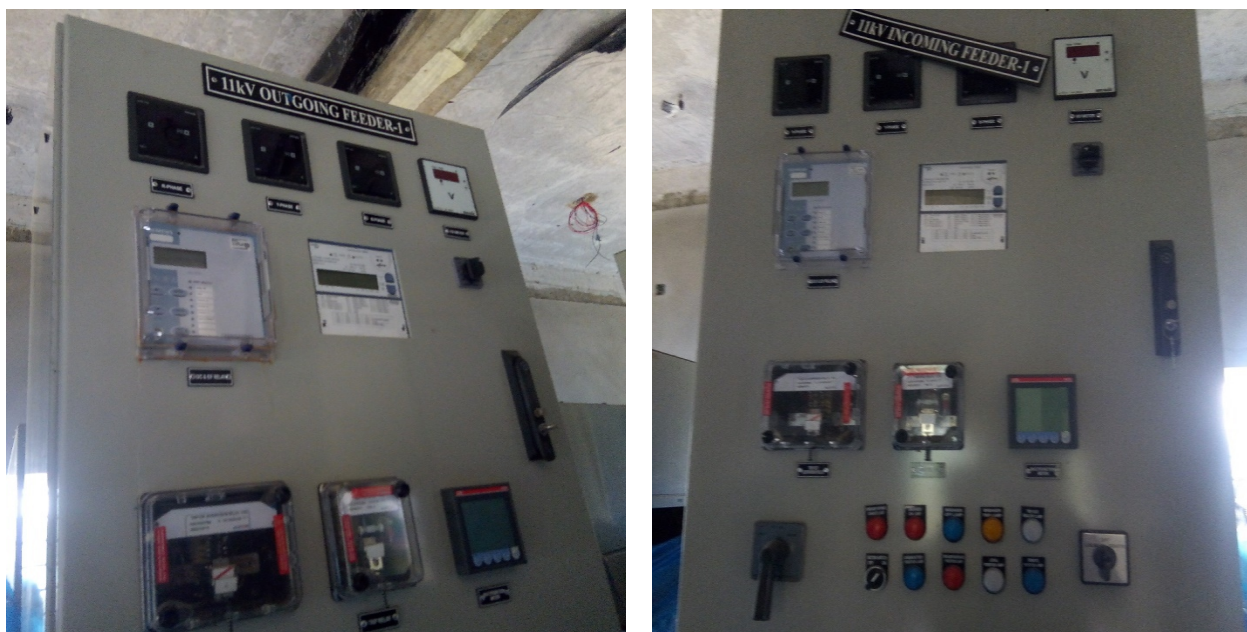
FIGURE 6: INDOOR COMPONENTS OF AN ELECTRICAL SUBSTATION
