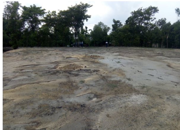
FIGURE 9: THE SUBSTATION SITE HAS BEEN RAISED ABOUT 5 FEET HIGH BY FELLING EARTH MATERIAL
